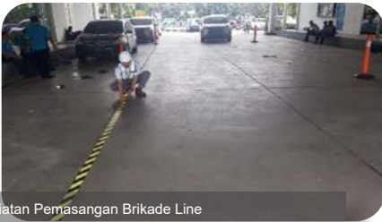
Kegiatan Pemasangan Brikade Line Line Bricade Installation Activities
